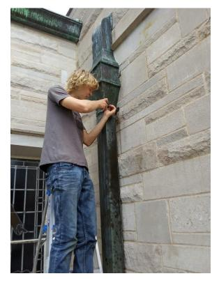
After the clean-out, Charlie refurbished the original bracketing that was barely holding the downspout to the side the building. Ready for the next 60 years!
